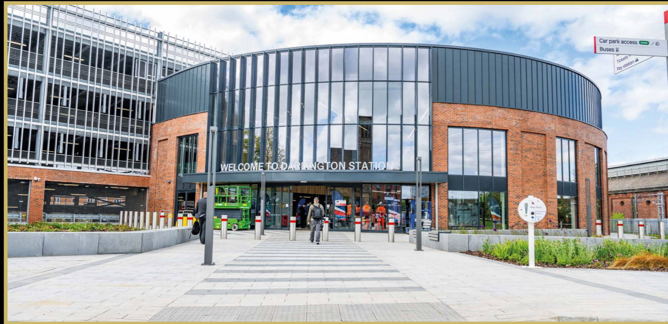
The new entrance to Bank Top Station.
